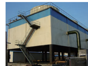
Steel structure cooling tower
