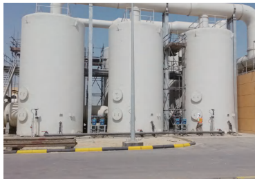
Vertical FRP storage tank Specification: DN100~DN4200、0.5~160m3
