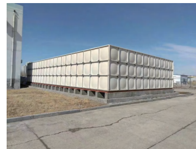
FRP Water Tank
