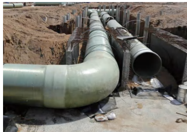
FRP pipe Specification: DN50~DN4000mm、PN0.1~3.2MPa、SN1250~SN20000N/m2
