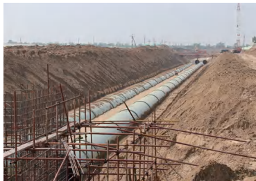
FRP pipe with sand Specification: DN10~DN3000mm、PN0.1~2.5MPa、SN1250~SN20000N/m2
