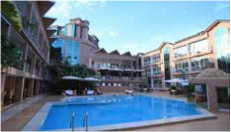
Location: Kigali, Rwanda Passenger elevator
