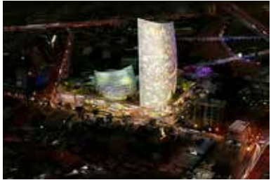
Location: Addis ababa, Ethiopia Passenger Elevator -2units Escalator -4units
