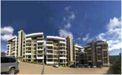
Location: Nairobi, Kenya Passenger Elevator -4units
