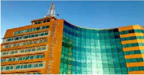
Location: Mogadishu, Somalia Passenger Elevator -4units
