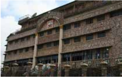
Location: Lagos, Nigeria Passenger elevator
