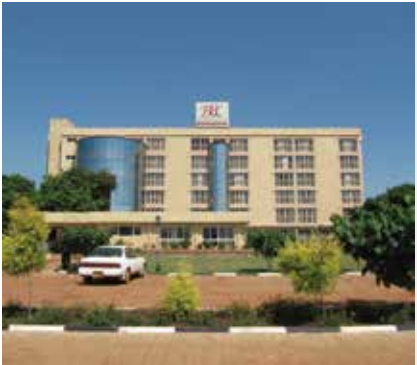
Location: Kampala, Uganda Passenger elevator
